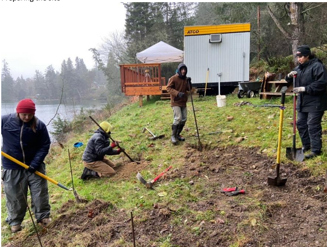
Preparing the site
